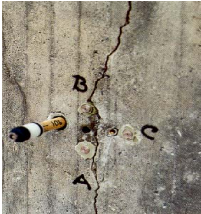
Fig. 11: location for expansion and humidity measurements, Elgeseter bridge.
